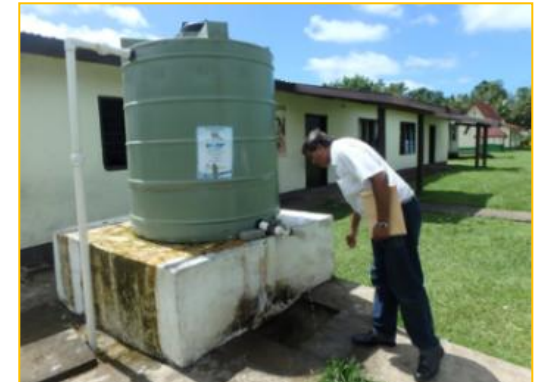
BALANCE Tank : over-flow to keep gentle flow for EPS
