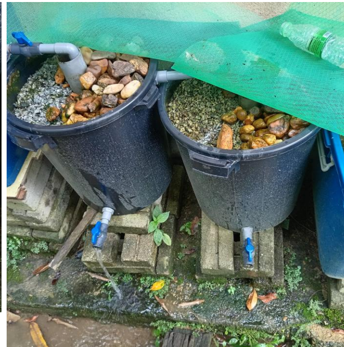
Backwashing up-flow roughing filter ⑧-163
