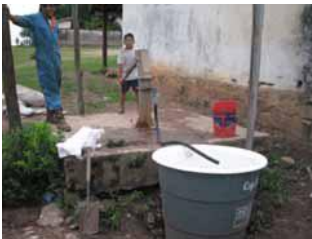
Pump for groundwater and source water tank
