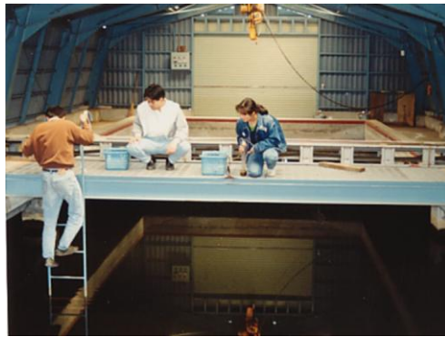
Covered filter: Iizuna, Nagano, Japan from 1974(S49).
