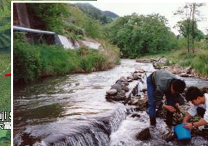
New intake of surface water for Someya WTP from 1953.
