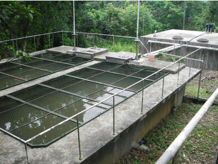
To protect against fallen leaves and branches, we covered it with wire mesh.
