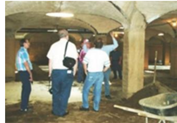
Covered filter from 1849, at Albany, NY, US Microscopic organisms play an active role in the covered filter.
