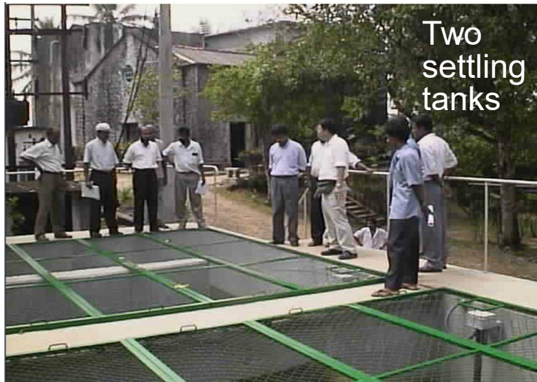
Turbid matter reduction by Settling tank and URF without chemicals.
