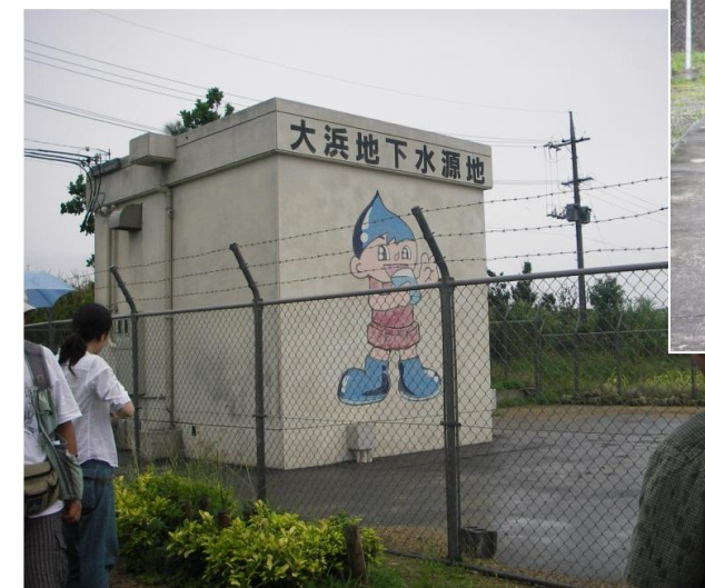
Pump station for underground water
