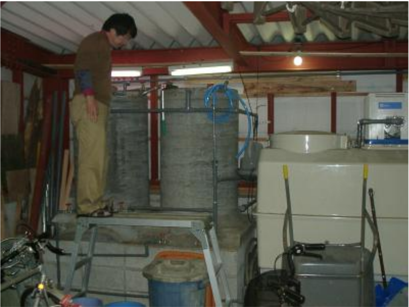
Final treatment of slow sand filter is in his garage.
