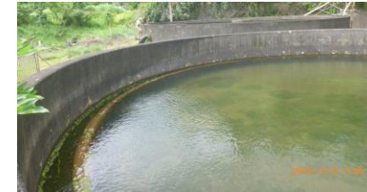
Up-flow Roughing filter:
