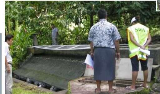
Intake Bar Screen filter
