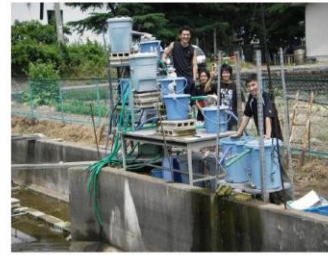
Multiple Roughing Filters to eliminate SS from an irrigation canal water.
