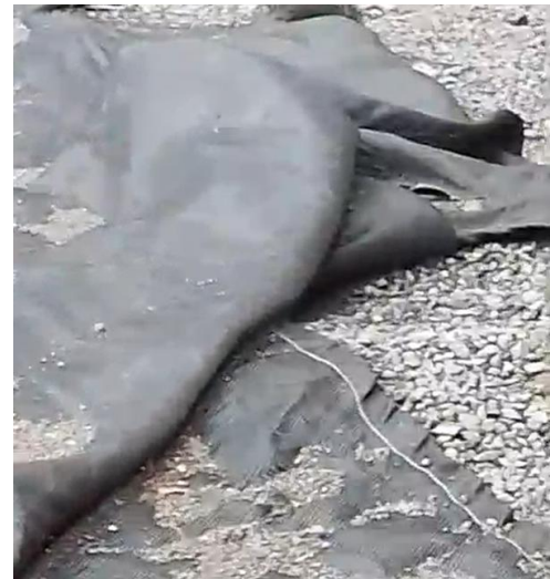
Cloth covered gravel layer.
