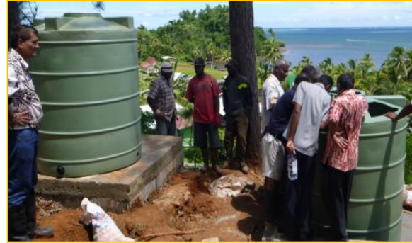
URF: Up-flow Roughing Filter
