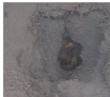
Accumulated mud on the gravel layer.
